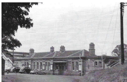
A view of the main station seen from the station drive, about 1960. Photo credit M.J. Lewis
